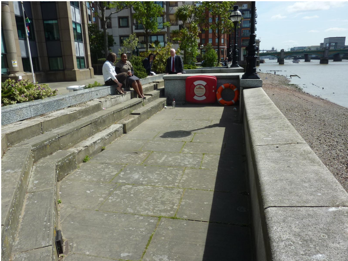
Existing Planter adjacent to the Riverside Wall
